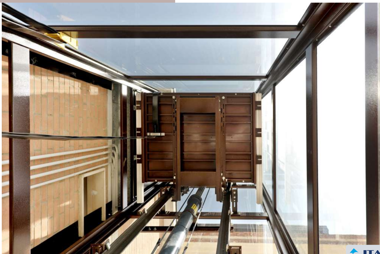
ARCATA E PEDANA VERNICIATE RAL CAR FRAME AND PLATFORM PAINTED RAL
